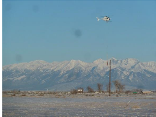
Conductor stringing with helicopter
