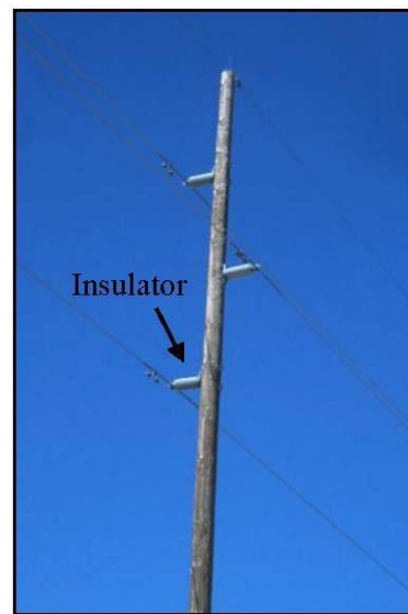
Post-mounted insulators
