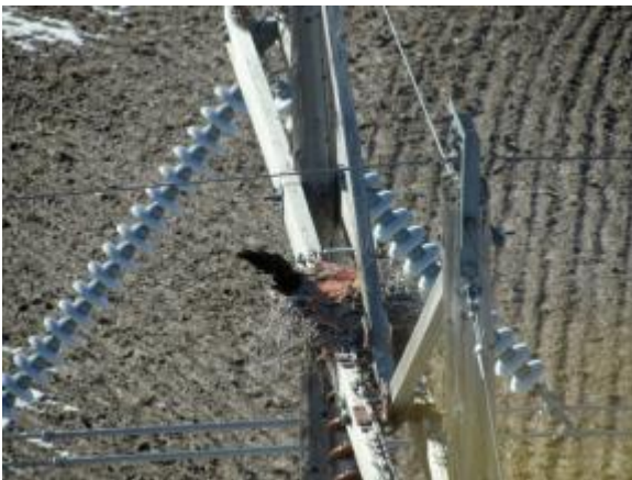
Common raven nest on transmission pole with spike discouragers.
